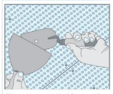
Fill screw heads with Knauf Snowboard-Finish using a Jet Trowel.
