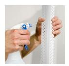
Using a spray bottle or pump sprayer, apply water liberally to the adhesive side of Gyproc AquaBead with clean, ordinary tap water, The warmer the water, the faster the activation.
