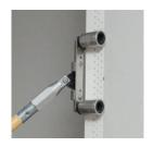
Press firmly by hand or with a roller, ensuring good contact between the flanges and the plasterboard.
