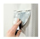
The Gyproc AquaBead corner can be filled after 30 minutes using Gyproc Joint Filler or Gyproc Joint Cement
