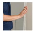
After applying water, allow 15 - 60 seconds for the adhesive to become sticky.
